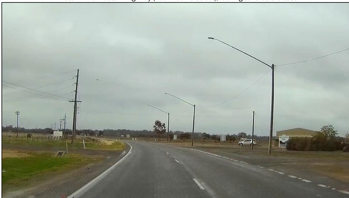
Photo 1: Mid-Western Highway (near Bourke Street), looking towards the east
